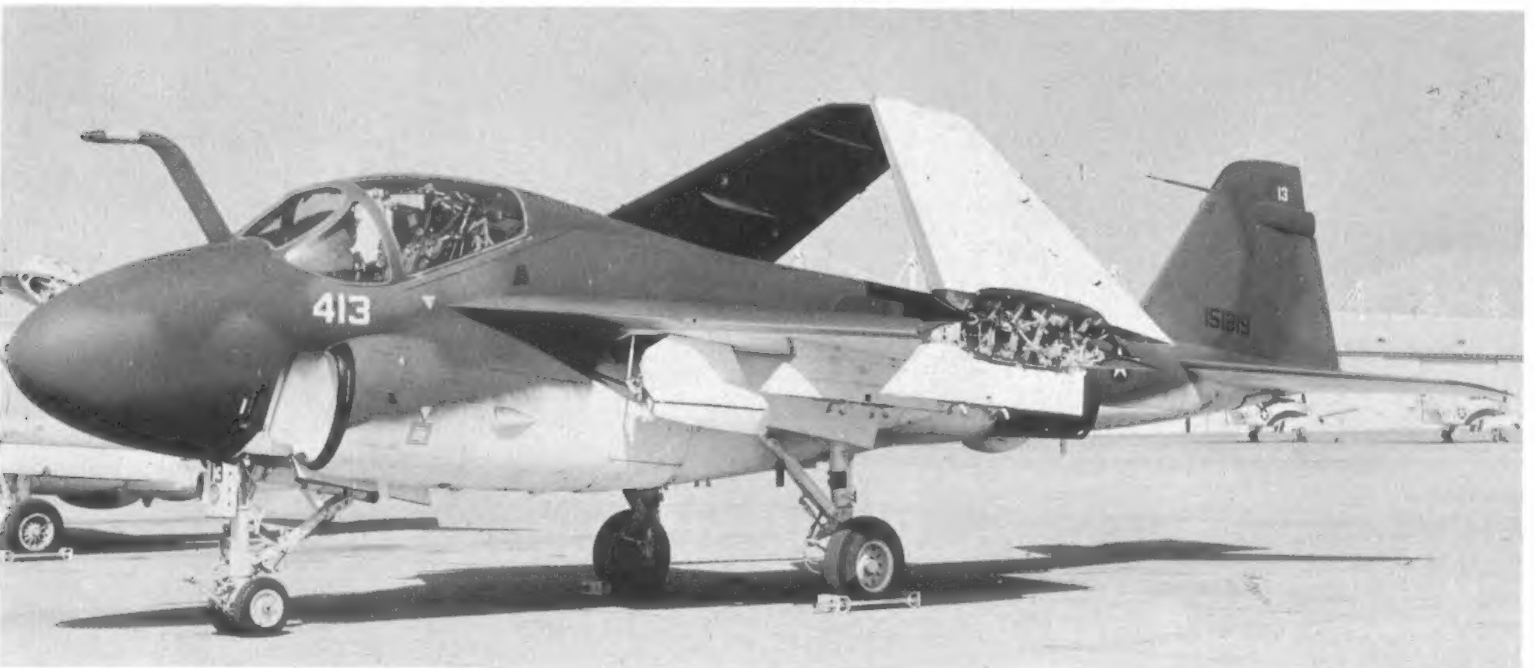
Camouflage evaluation, spring 1966. Upper surfaces were dark (almost black) green and deep blue while under surfaces remained flat white. National insignia was reduced in size. A-6A (BuNo. 151819) was assigned to VA-65 Tigers. Photo at NAS Lemoore, Calif. (Photo: Unknown)
